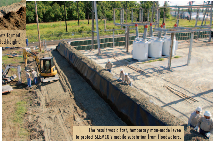
The structure was covered with liner. Seams were sealed and additional limestone was added to secure the liner.
