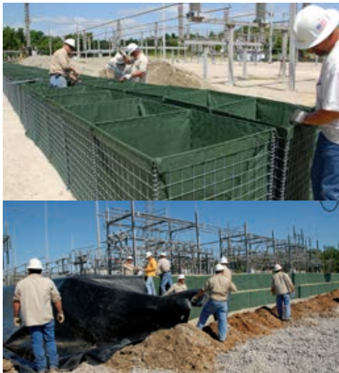
Within 34 hours, SLEMCO personnel ensured the protection of service to two towns, thousands of consumers and a refinery by building a six-foot levee around our Krotz Springs substation.
