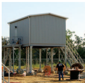
The rebuilt Esther substation (photos below) will be online by year's end. Along with the Erath (above) and Cow Island substations, it was part of a $6.6 million project begun in 2010 to raise substations above hurricane floodwaters.
